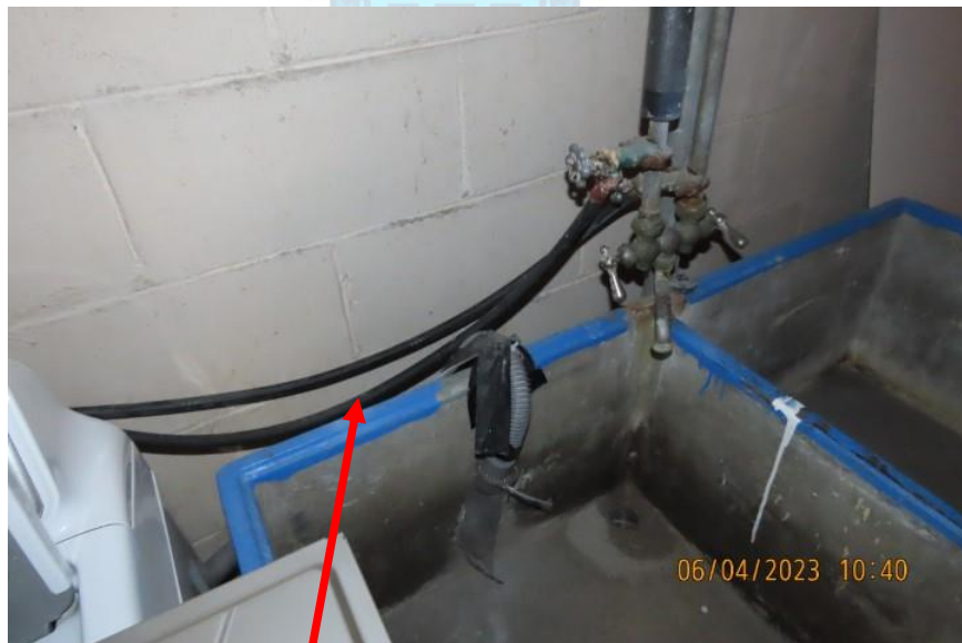
Black rubber hoses have a low psi strength
