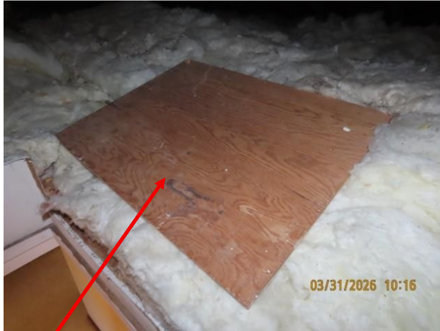
The attic hatch should be insulated and weather stripped
